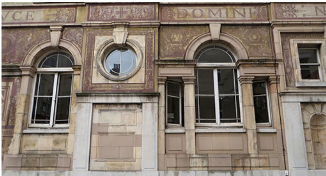
Carter Lane YHA, formerly St Paul's Choir School. Note the masonry using red sandstone below the windows.
