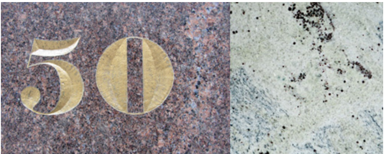
Windsor House. Left; Dakota Mahogany granite; Right; Kashmir migmatite. Garnets are 2-5 mm diameter.
