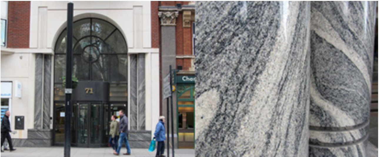
71, Victoria Street, right; details of the gneissic banding on the columns.
