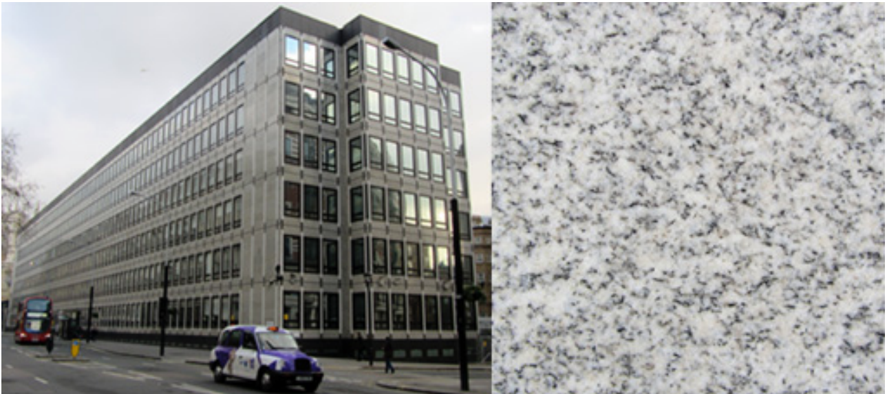
Department of Business, Innovation and Skills clad with white Støren trondhjemite, right.
