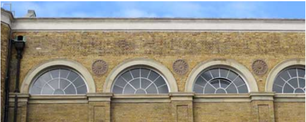
The 1849 Library Extension. Note the yellowish stones framing the windows in contrast to the white Portland Stone along the roof line.
