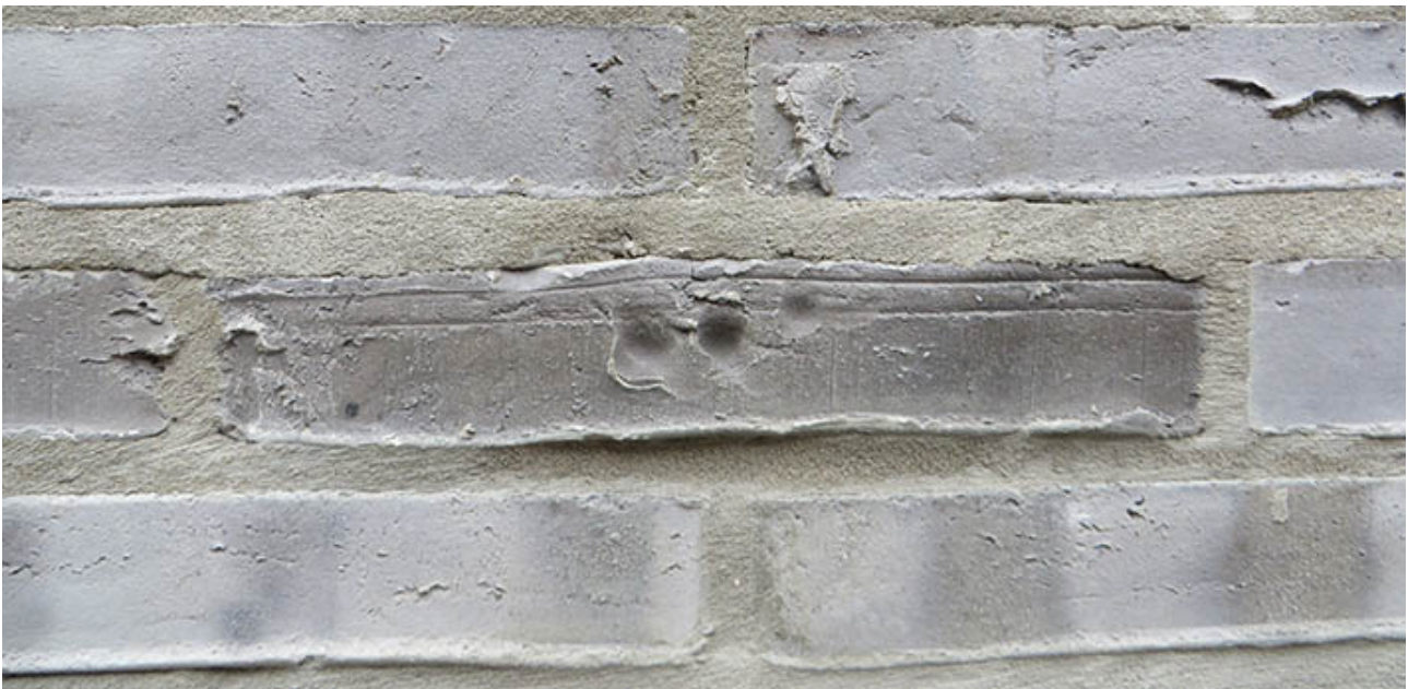
Above: The Gordon Street Klinker bricks used at The Bartlett School of Architecture. Note the fingerprints and the grey colour denoting a low iron content. Each brick is 290 x 52 x 70 mm.
