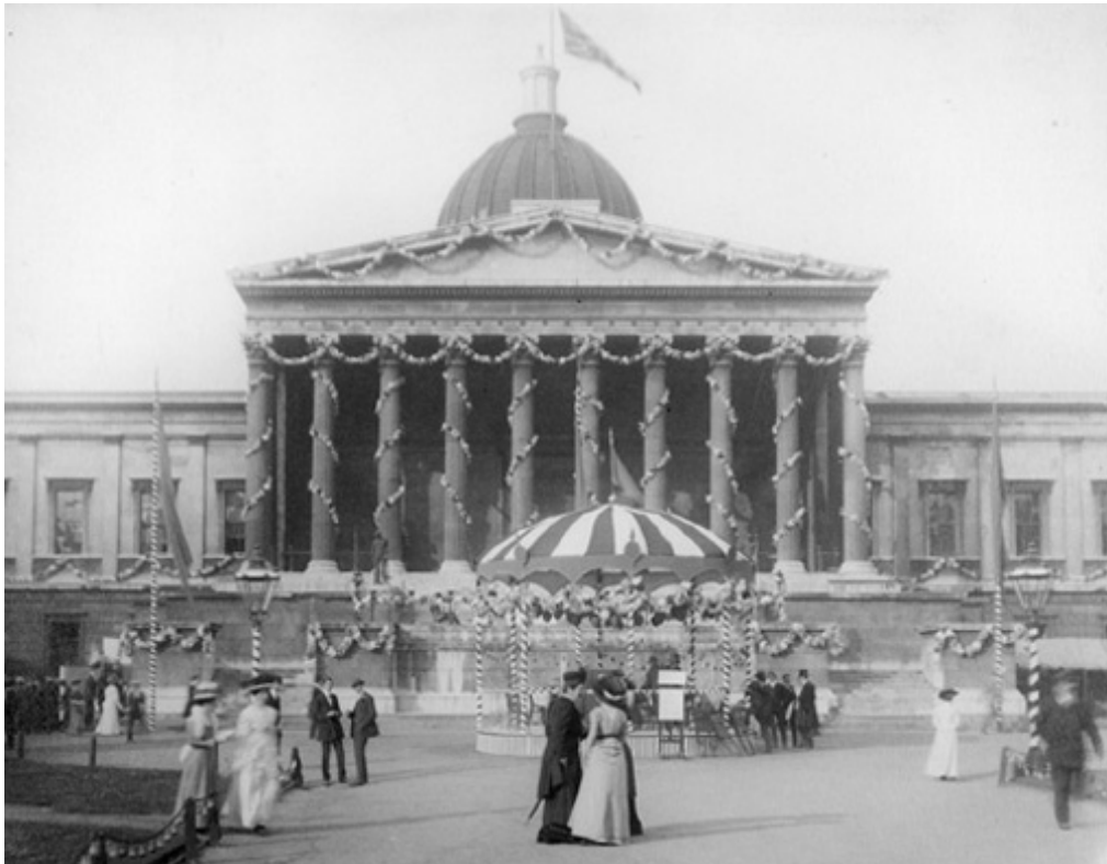
The Main Quad during a fete in 1909. The dark colour of the Portland Stone is obvious and streaks can be seen along the front. Compare with the frontispiece photo, taken in Autumn 2013, following steam cleaning earlier in the year.
