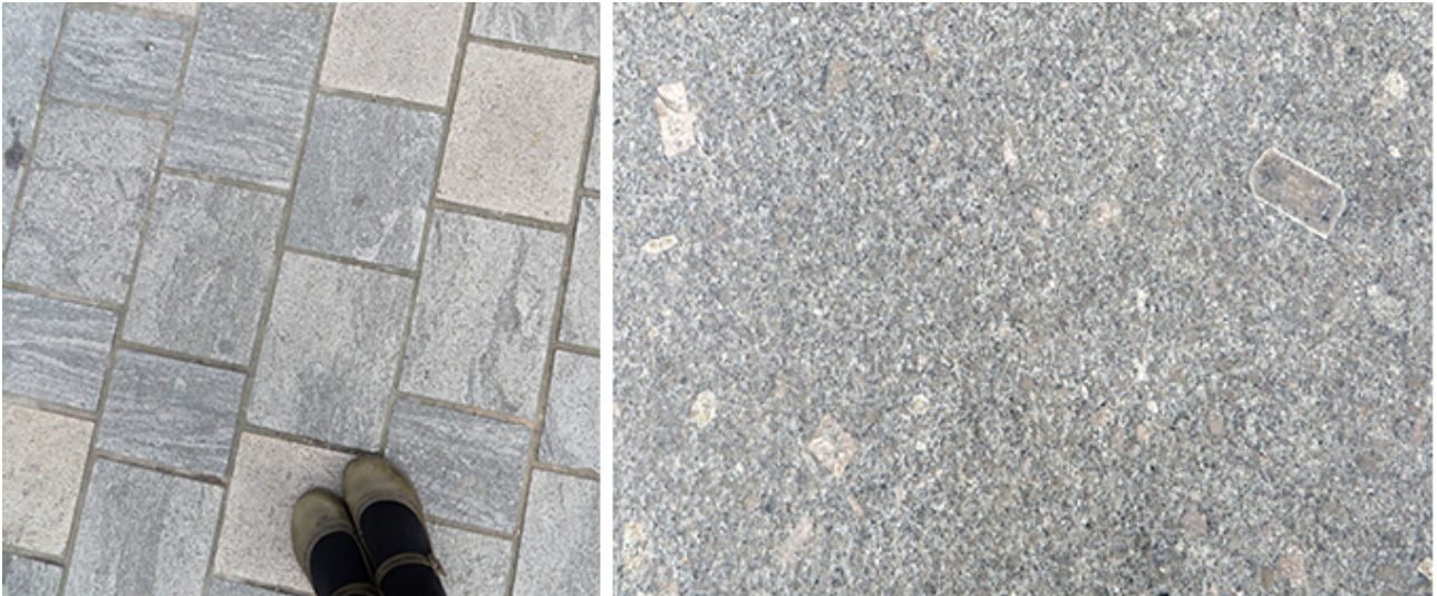
Left: granite and gneiss setts, Byng Place and right: porphyry granite in Torrington Square, field of view 60 cm.
