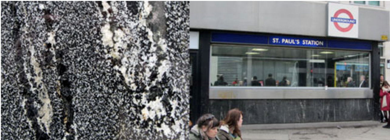
St Paul's Station Kiosk, with left, close up of 'Tatra B' gneiss.
