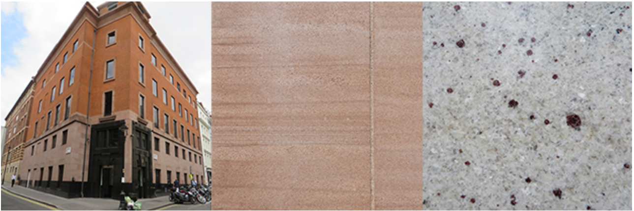
Above left; 53-59 Chandos Place; middle, detail of the red sandstone and right; detail of the garnet-bearing meta-granite at 65 Chandos Place.
