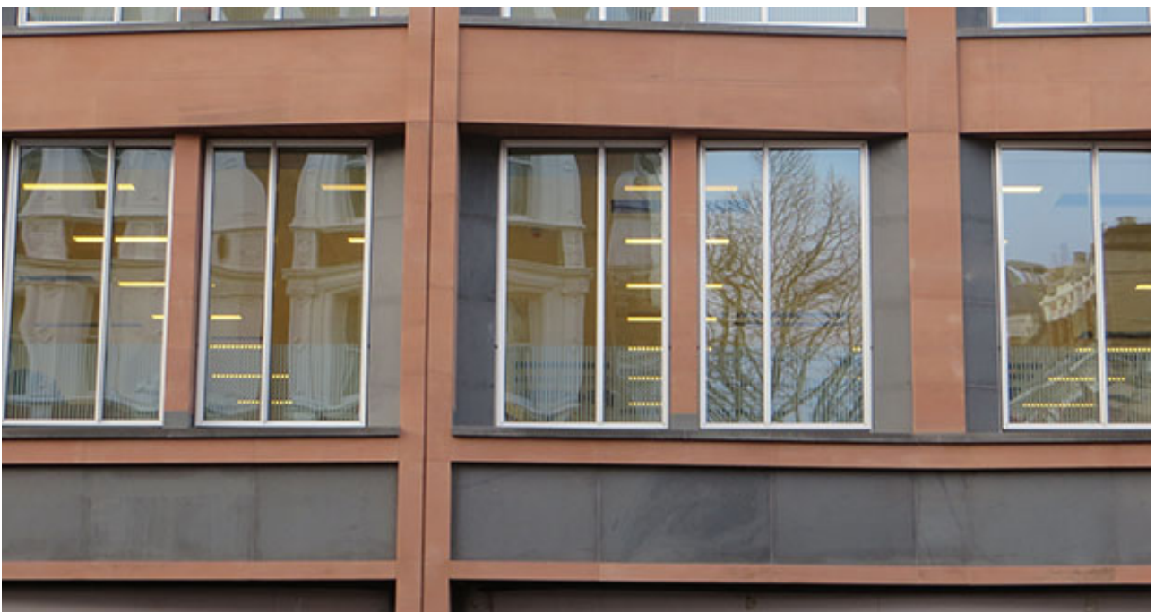
Locharbriggs Sandstone and Etna Lava Stone cladding on the façade of 131, Sloane Street.
