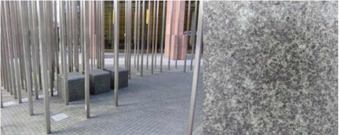
Left: Regent's Place Pavillion. Right: the green gabbro used on the seating.
