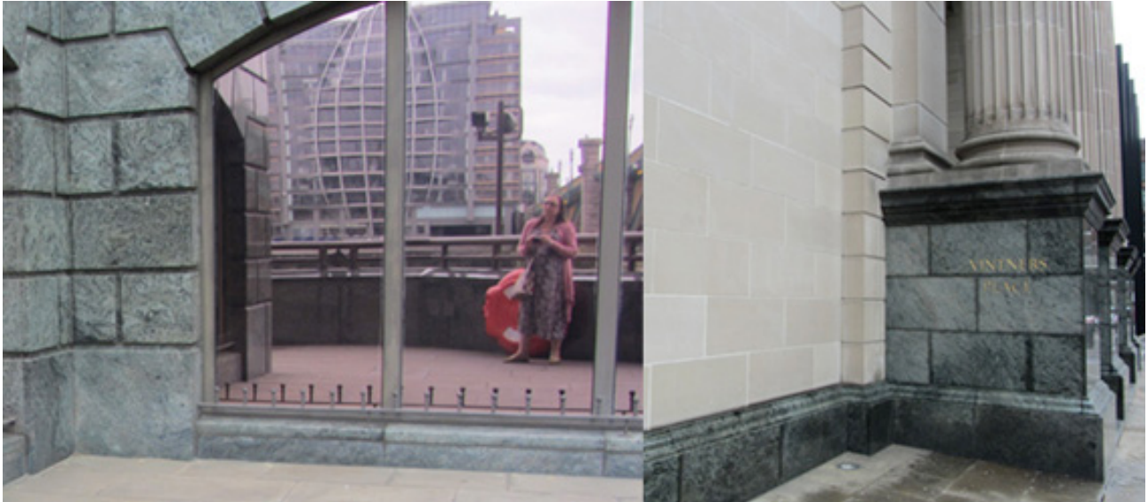
Vintner's Place: Left, Verde Candeias clads the foundation courses of the building. Right, Verde Candeias with Indiana Limestone above.
