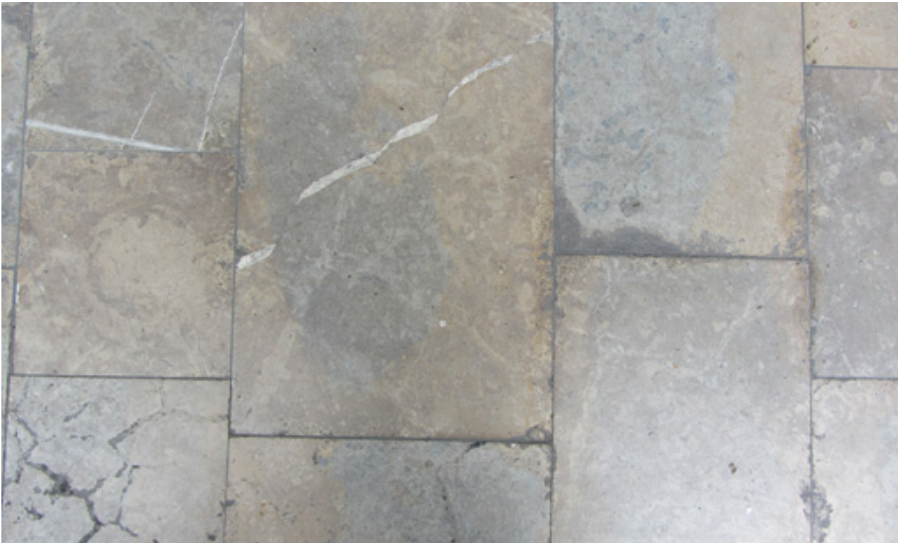
Purbeck Cap paving at Thames Court.
