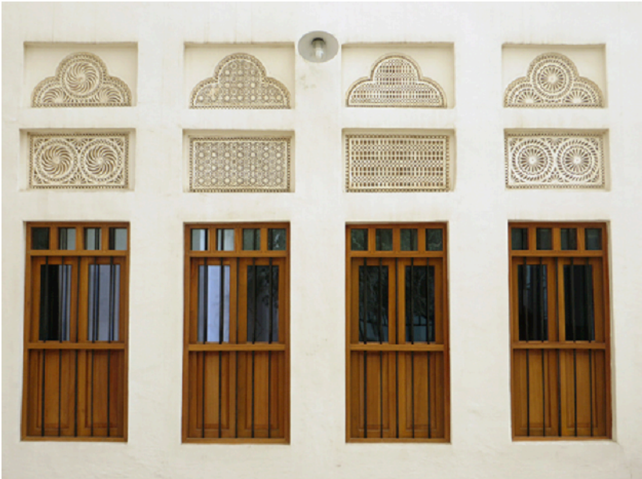
The Radwani House with traditional gypsum grills above the windows.
