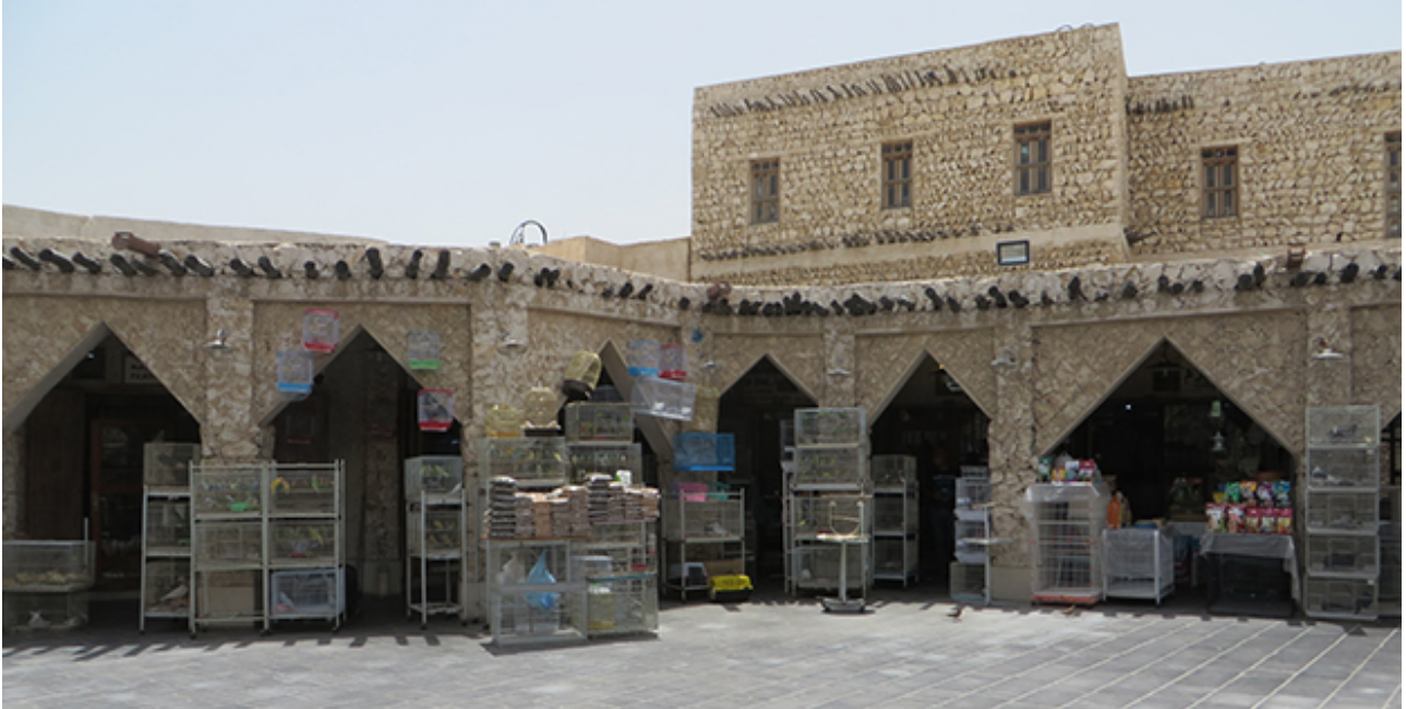
The Bird Market in Souk Waqif. Rubble masonry construction, with wooden poles supporting the ceilings.
