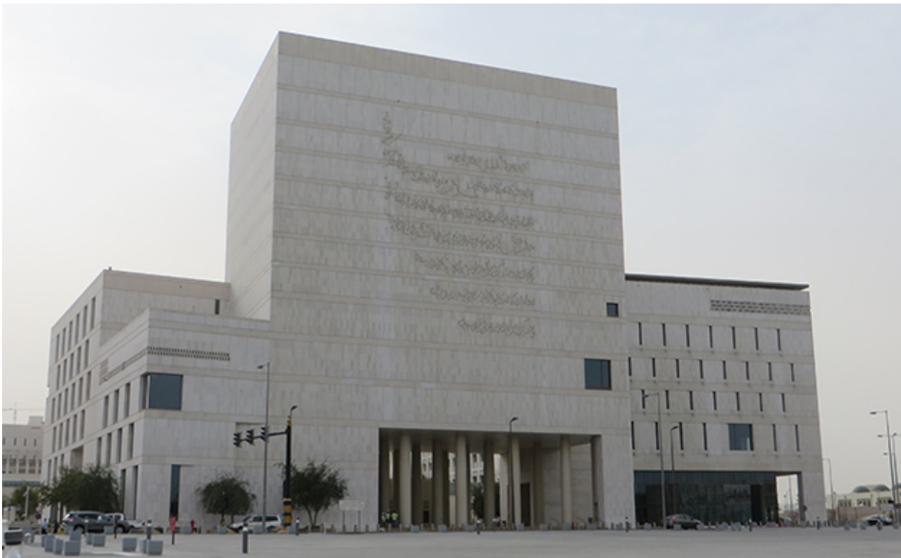
The National Archives in the Msheireb Downtown Complex, clad in Oryx Limestone from Oman.
