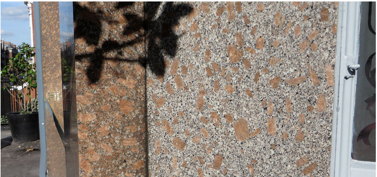
Dark and Light Shap Granite, The Crown & Sceptre, 86 Great Titchfield Street W1.
