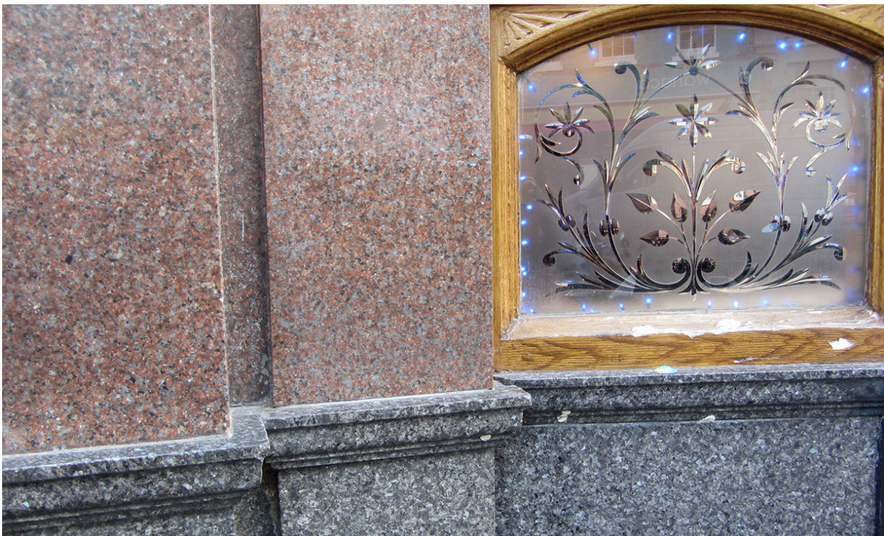
Fitzroy Tavern, 16 Charlotte Street W1T 2LY; contrasting Scandinavian granites, Swedish Balmoral and larvikite
