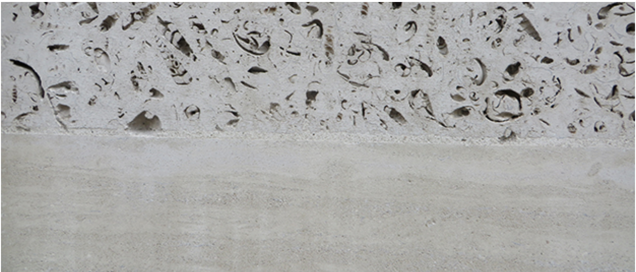
Above; a block of Roach placed on top of cross-bedded Whitbed at 23 King Street, W1 .
