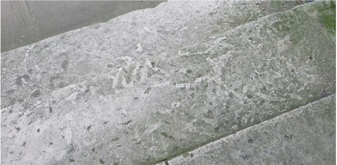
Above: Thalassinoides burrows in Portland Stone Whitbed. The steps of the Kathleen Lonsdale Building at University College London .
