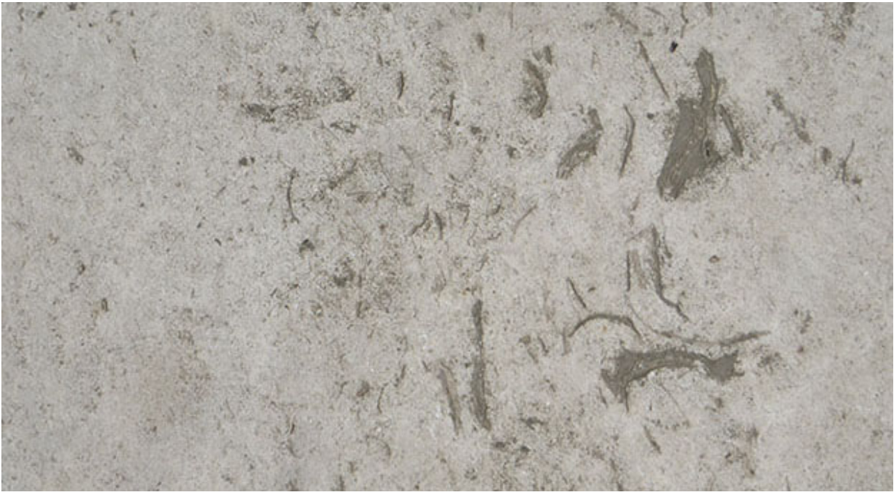
Portland Whitbed with oyster-shell fragments sub-aligned parallel to bedding, which runs vertically across this image.
