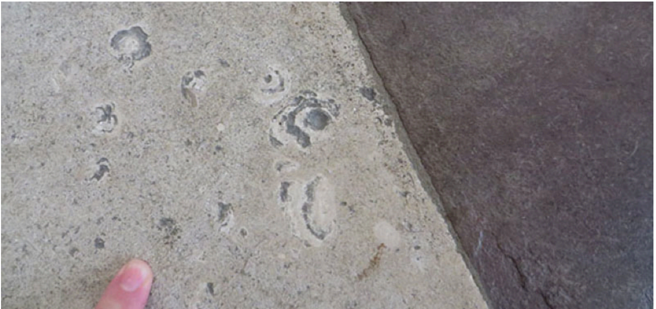
Detail of the foyer paving; on the left of the image, the white Portland Stone contains debris of the alga Solenopora portlandica . Liver-coloured red sandstone is on the right.
