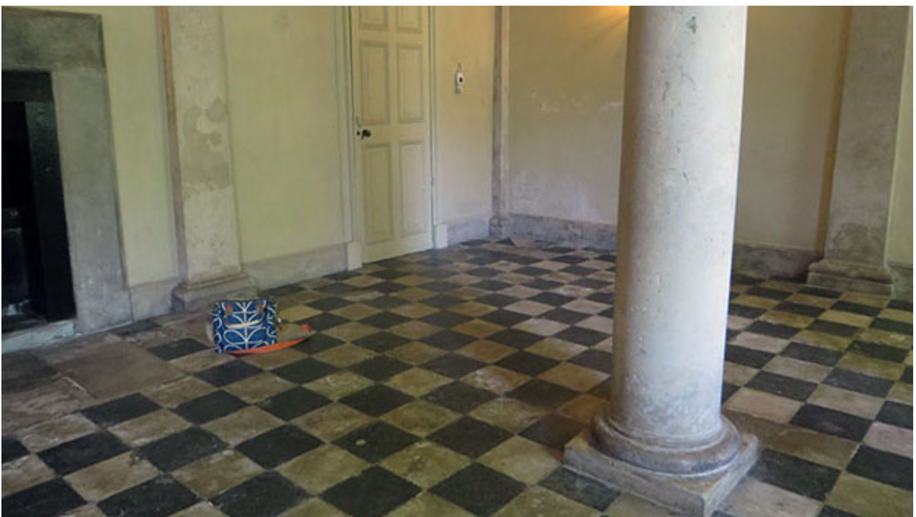
The Tudor Floor in the Servants Hall. The Portland Stone Columns are later.
