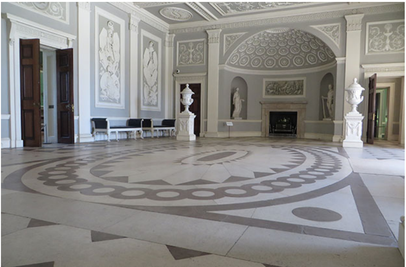
The foyer of Osterley Park House with the floor paved in red sandstone and white Portland Stone. Note the fireplace in the apse. The stone used for this has not yet been identified, but it is possible that it is a compact, fine-grained variety of Bath Stone.
