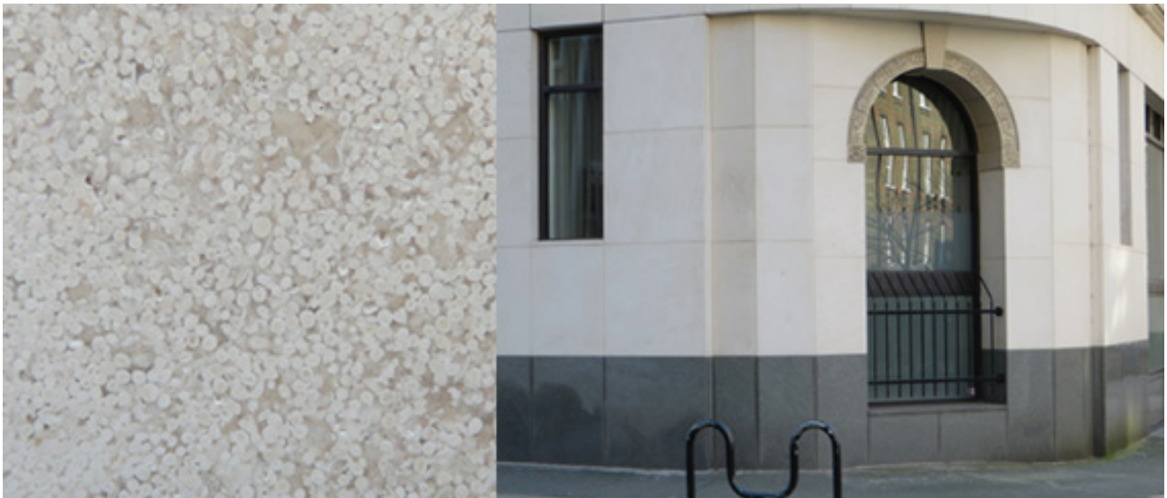
Left; oosparite limestone, each ooid is approximately 1 mm in diameter. Right; 21-27 Lamb's Conduit Street.
