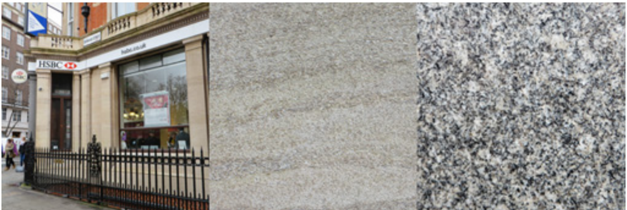
Left; HSBC Bank on Bernard Street; Centre: cross-bedded, coarse grained, Carboniferous Millstone Grit Sandstone; Right: Cairngall Granite on the door frame.
