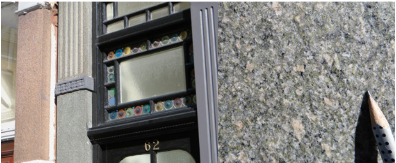
Left: pilasters of pink Peterhead Granite and the grey-green granite at No. 62; Right: the grey-green granite.
