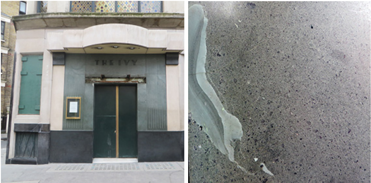
Above left; entrance to The Ivy on west Street. Right; Lake District Green Slate with a rip-up clast of fine grained ash.
