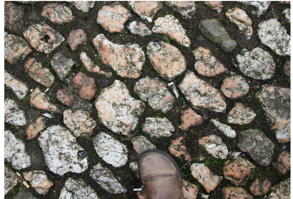
Veinstone, the waste product of metal mining which makes hard-wearing cobblestones that are used for paving in various localities in the town of Helston. It is best seen at Five Wells and outside the Band Hall on Church Street.
