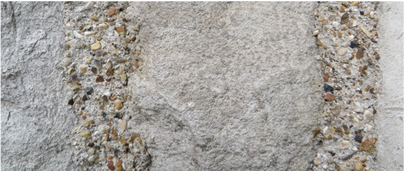
Above: The River Thames seeps between the stones of St Augustine's Tower; flint-rich mortars cementing Kentish Ragstone.
