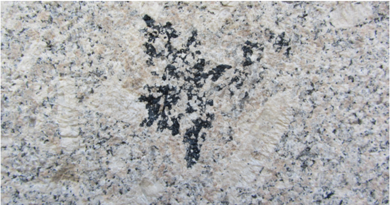
Dartmoor Giant Granite in the foundations of Goldsmith's House, FOV 20 cm.
