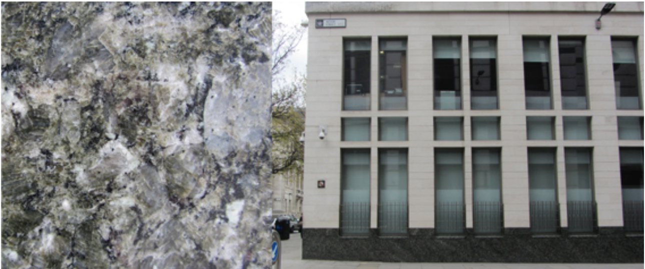
31 Gresham Street. Left: the coarsely crystalline texture, with large grey-blue microcline feldspars. Right: strong foliation on the charnockite can be seen in the foundations. Field of view is ~ 8 cm.
