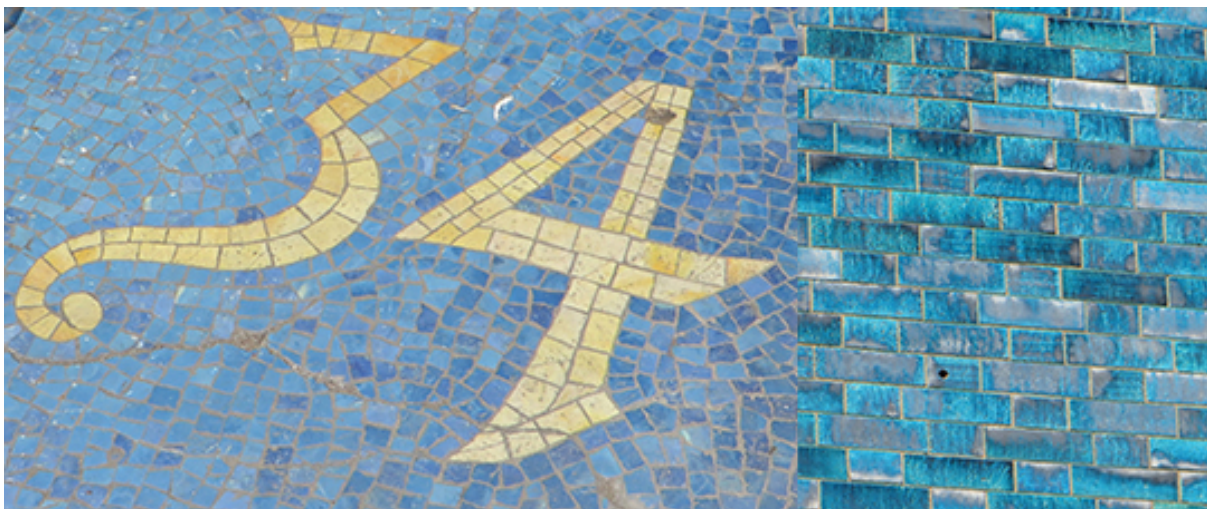
Left; Mosaics in the doorway of Radiant House, Right: the blue faience tiles.
