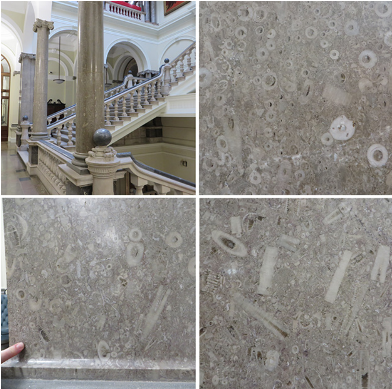
Figure 7. The 1 st floor of the Muses Staircase with pillars of spectacular crinoidal marble from Ricklow Quarry in Derbyshire.
