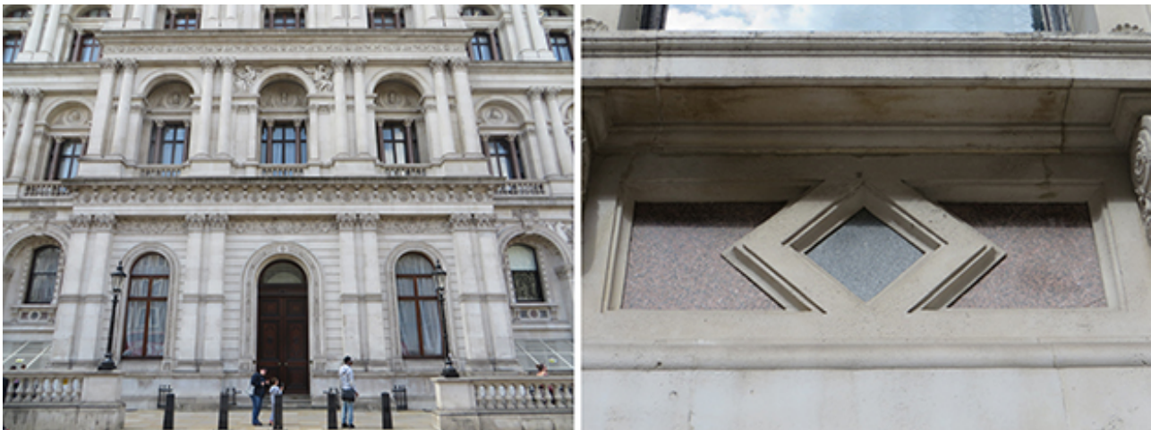
Figure 1. The Exterior of the Foreign, Commonwealth and Development Office and detail of decorative panels using pink and grey Aberdeenshire granites.
