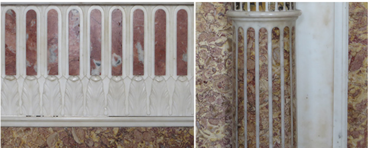
Figure 10. Detail of the fireplace in the Locarno Suite Conference Room. White Carrara marble, red Rosso Verona and a red and yellow Brocatello.
