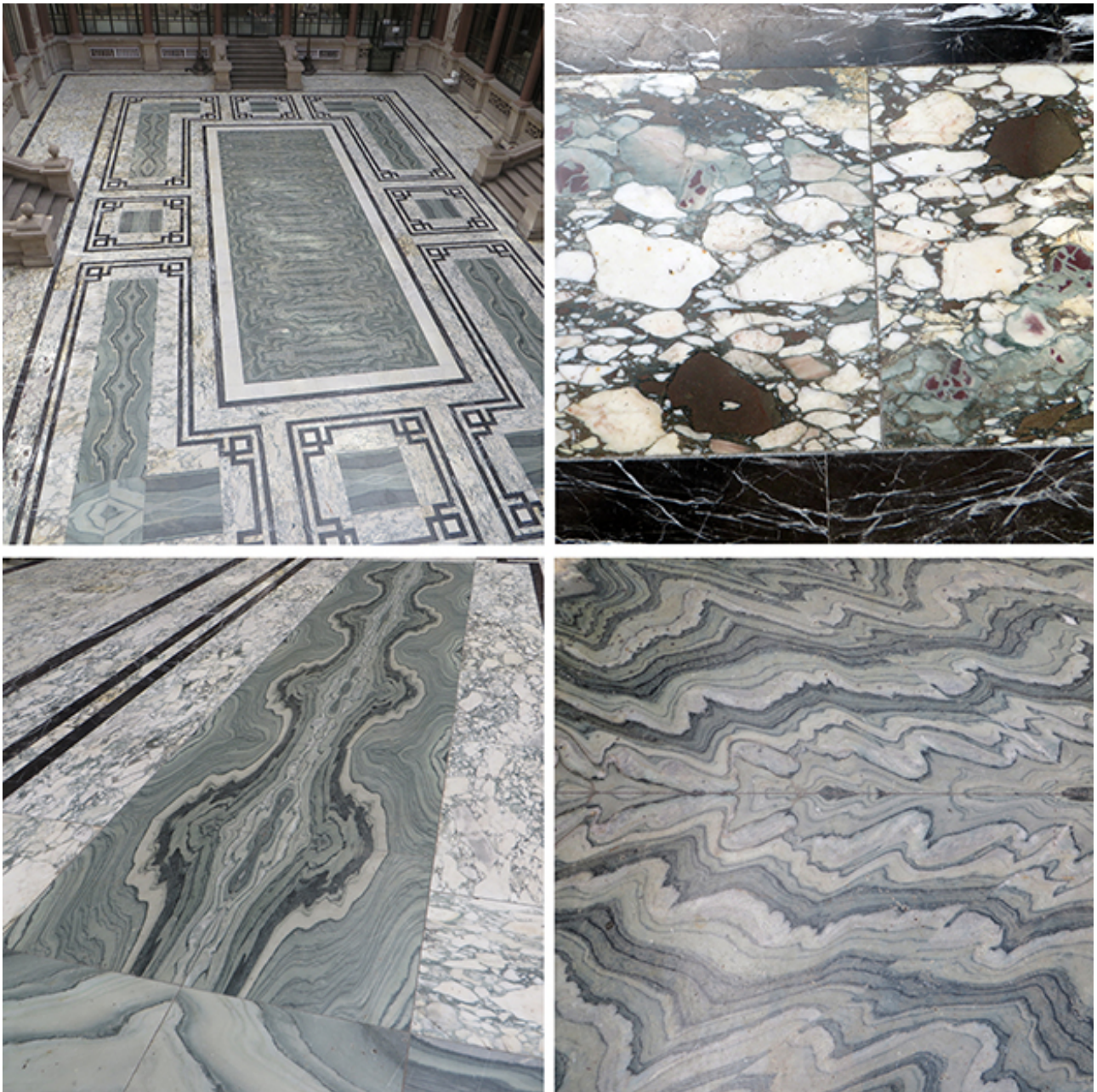
Figure 6. The Durbar Court and detail of the marbles used. Top right, Carrara breccias with black Buckfastleigh Marble and below, book-matched Cipollino Marble.
