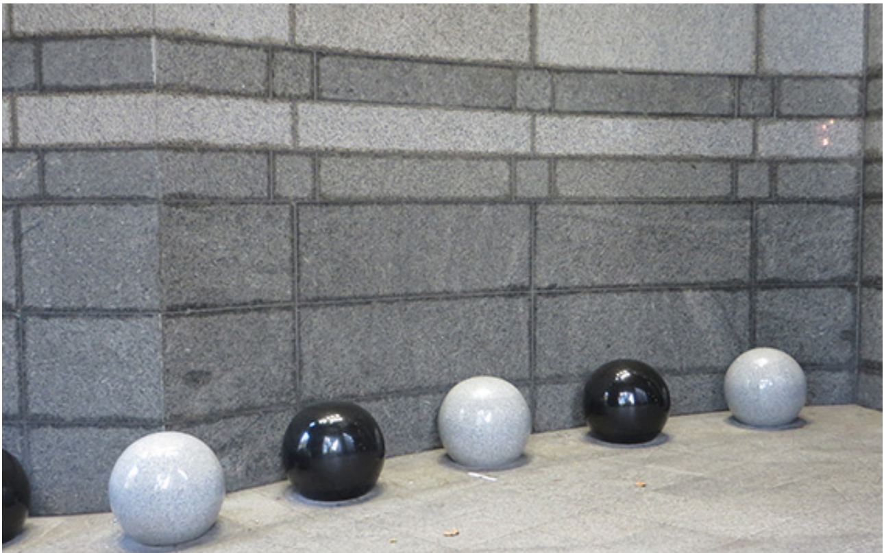
1, Embankment Place with the newly installed granite balls (October 2014).
