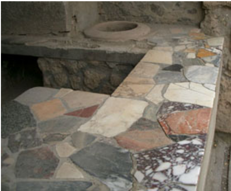
Left: Thermopolion counter with slabs of stone including marmor Phrygium or Docimenium (Pavonazetto) in the bottom right corner. This is a marble breccia from Iscehisar, ancient Dokimeion in Turkey; an Egyptian gabbro at the far left; various pieces of marmor Luculleum (Africano) breccia from Teos in Turkey; yellow marmor Numidicum (Giallo Antico) from Chemtou in Tunisia; salmon-pink marmor Chium (Portasanta) from the Greek Island of Chios in the Aegean; pale yellow-pink Breccia Corallina, from Bilecik (ancient Bythinia) in Turkey. The white and grey marbles which could have been derived from Greece, Italy or Turkey. Also present on this counter is marmor Carystium.
