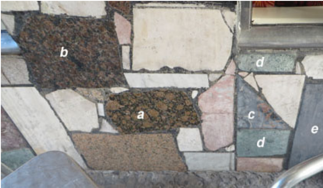
Lamb's Conduit Street façade; a). Baltic Brown, b). Indian Brown Granite, c). Portoro, d). green serpentinite, e). black limestone.
