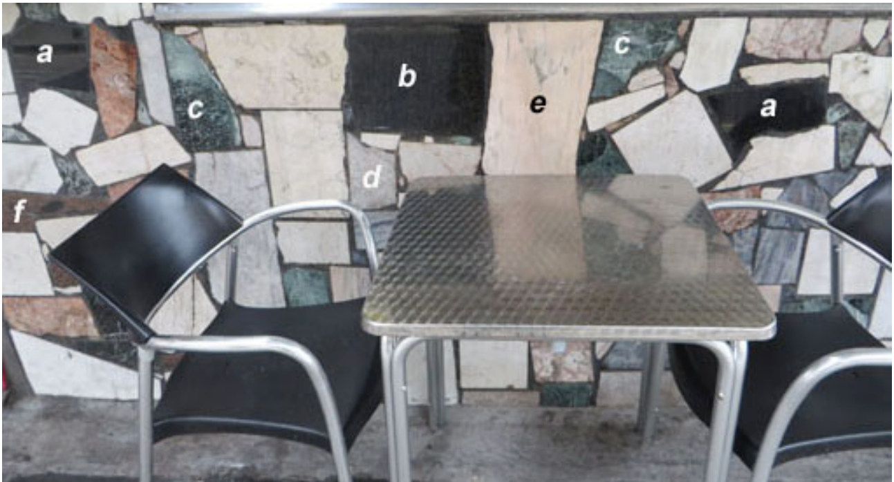
Rugby Street façade; a). Belfast Black, b). Rustenburg Bon Accord, c). green serpentinite, d). Napoleon, e). Rosa Portogallo.
