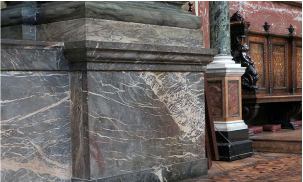
Plymouth Marbles in the plinths of the nave columns. The main section is Mill Quay Marble. The pattern of veining is very typical of that associated with the deformation of the Plymouth Marbles. Kitley Green Marble forms the uppermost layer visible here.
