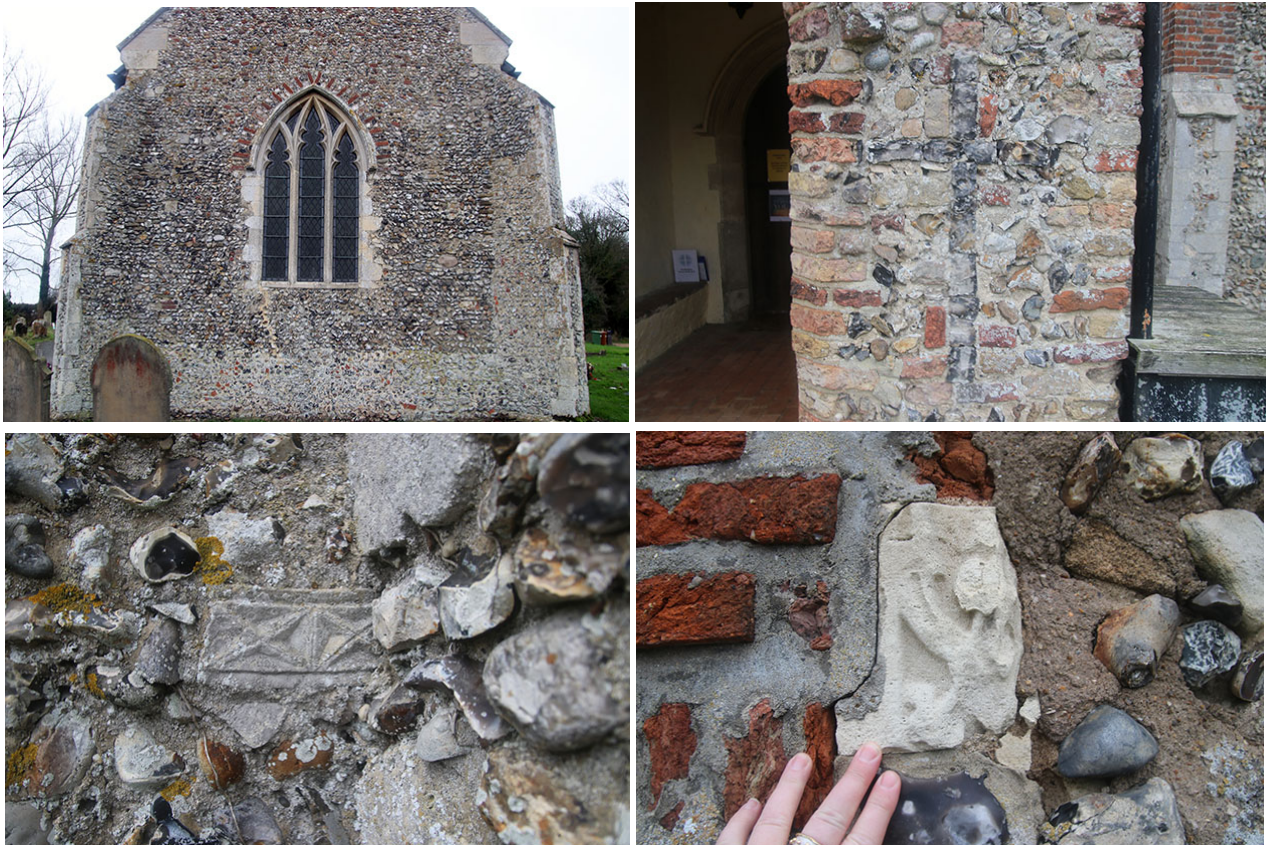
Top left: The east end of All Saints Church, Hemblington showing at least two phases of construction. Top right: flushwork flint crosses in the brick-built south porch. Bottom left: Carved spolia and rough flints in the walls. Bottom right: Carved spolia in Caen stone. This is the remains of a window sill which has been cut into by Tudor brick work (on the left of the image).
