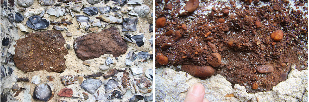
Left: Blocks of ferricrete at St Helen's Church, Ranworth. Right: the stone has variable texture and clast size/distribution. However, it is notably a bright. Brick red in colour.
