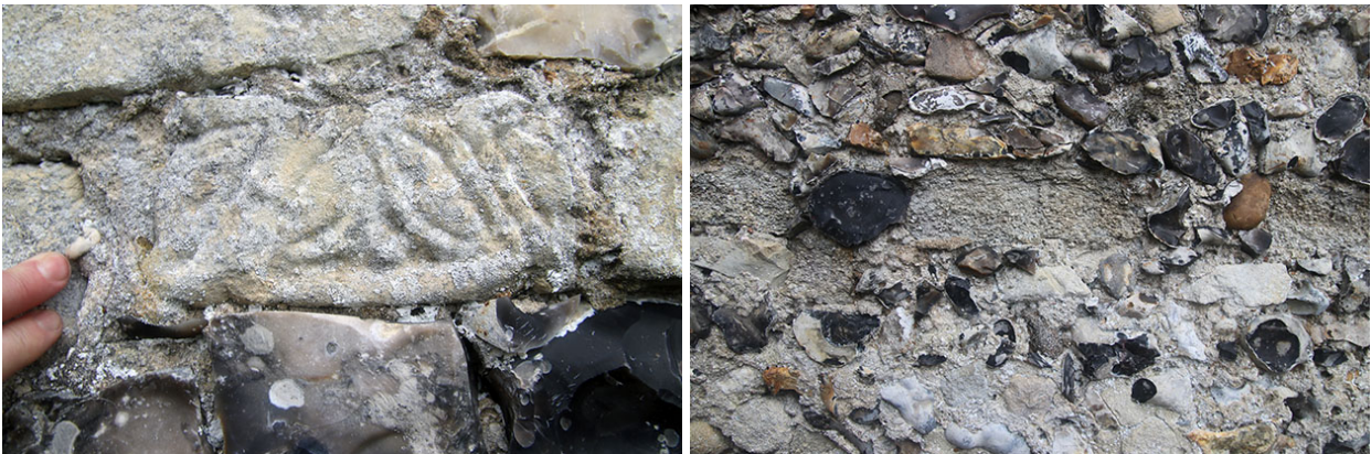
Left: St Mary's Church, South Walsham. Fragment of carved capital in Caen Stone used as spolia in the church's fabric. Right: slabs of Purbeck stone, weathering in a line across the centre of the photograph.
