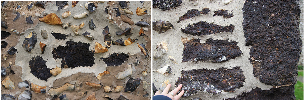
Left: Blocks of ferricrete along with unknapped, uncoursed flints in the south wall of St Peter's Church, Belaugh. These stones have been recycled into restoration phases. Right: Ferricrete used as quoins and ashlar on the NE corner of the church.
