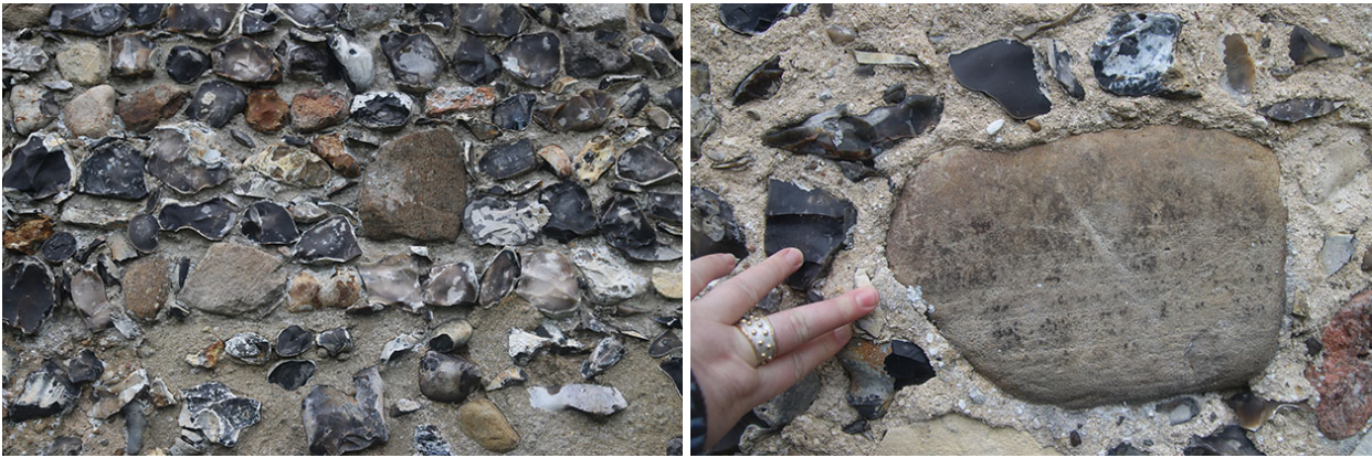
Left & right: Knapped, coarse flints with boulders of brown arenaceous sandstone at St Mary's, South Walsham. The photo on the right shows a boulder which may show evidence of glacial striae.
