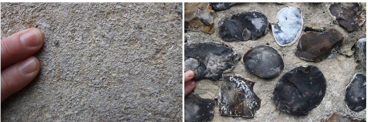
Stonework at St Lawrence's, South Walsham. Left: detail of Clipsham Stone dressings; this cross-bedded calcarenite is packed with shell fragments. Right: Knapped flint cobbles.
