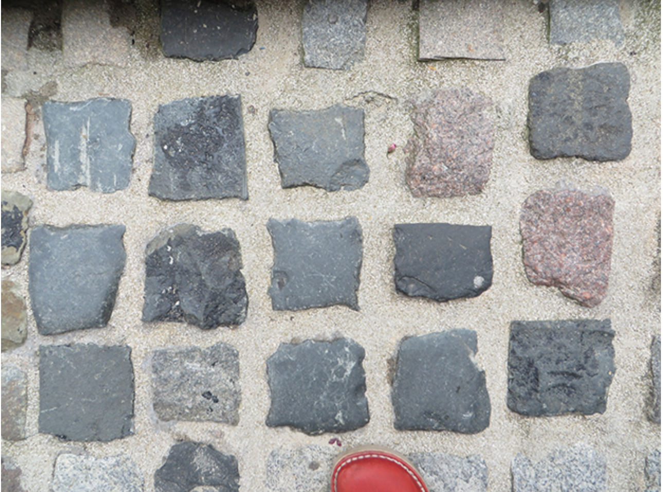
Reclaimed cobbles in Oozells Square. Dark grey cobbles are Whinstones, and some may well be Rowley Rag. The three pale grey and pink stones at the top right are Trefor Granite. The two red stones are Mountsorrel Granodiorite.
