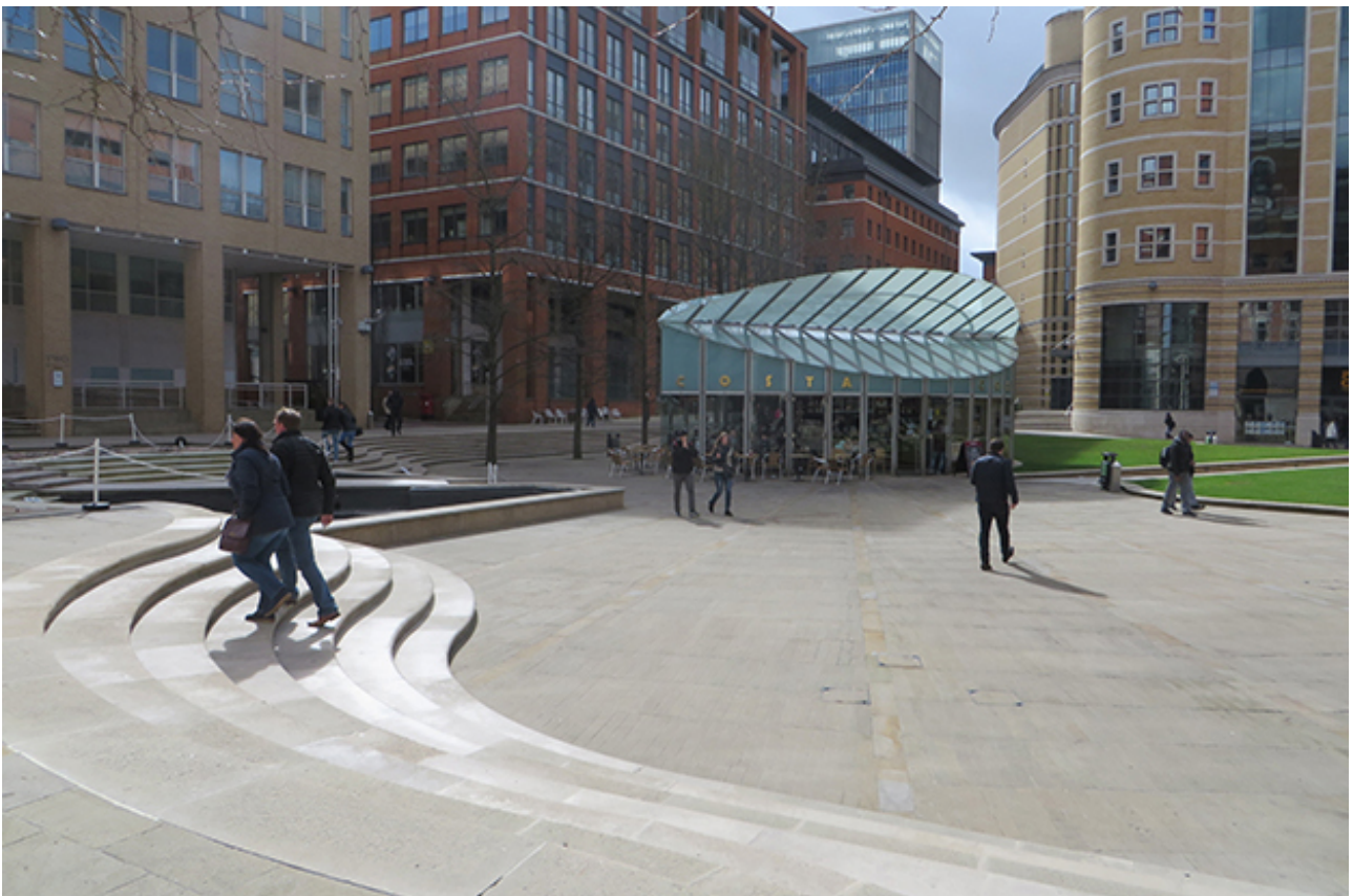
Brindleyplace; steps are of Portland Stone and the paving is York Stone, a Carboniferous sandstone.
