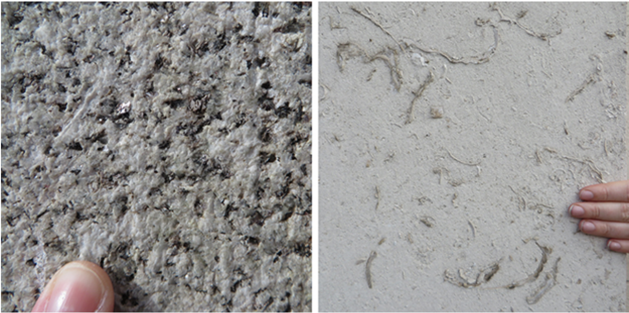
Cornish Granite with both muscovite and biotite mica (left) and Portland Whitbed with oyster fossils (right). This combination of stones is seen on the Hall of Memory, Baskerville House & the First Municipal Trading Bank.
